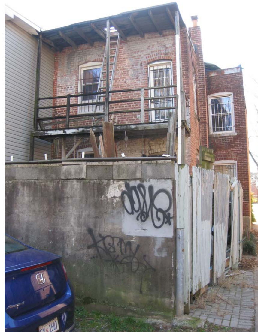
REAR OF 1005 P ST. NW
