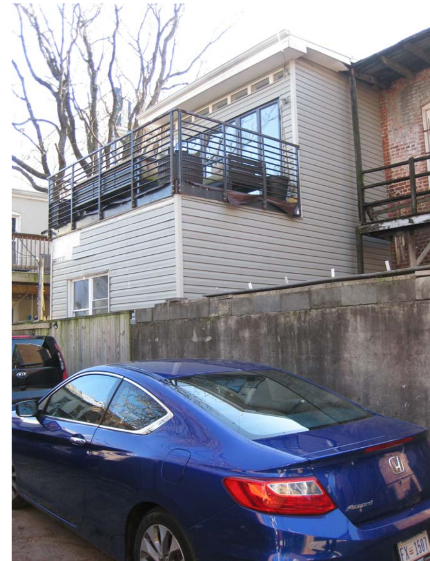
REAR OF 1003 P ST. NW
